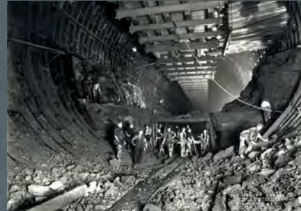
Hear how the tunnel was constructed.
